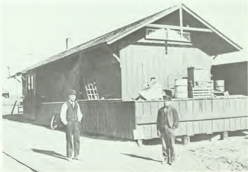
The Camargo, Oklahoma, depot is representative of the inexpensive standard wood frame structures utilized by the Wichita Falls and Northwestern Railroad at small way stations in western Oklahoma.
